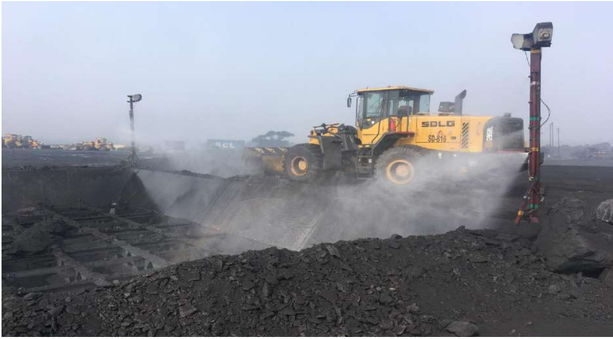
Photograph-1: Automatic mist type sprinkler near hopper
