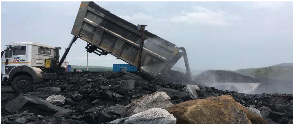
Photograph-3(b): Mist sprayng during unloading of coal at crusher
