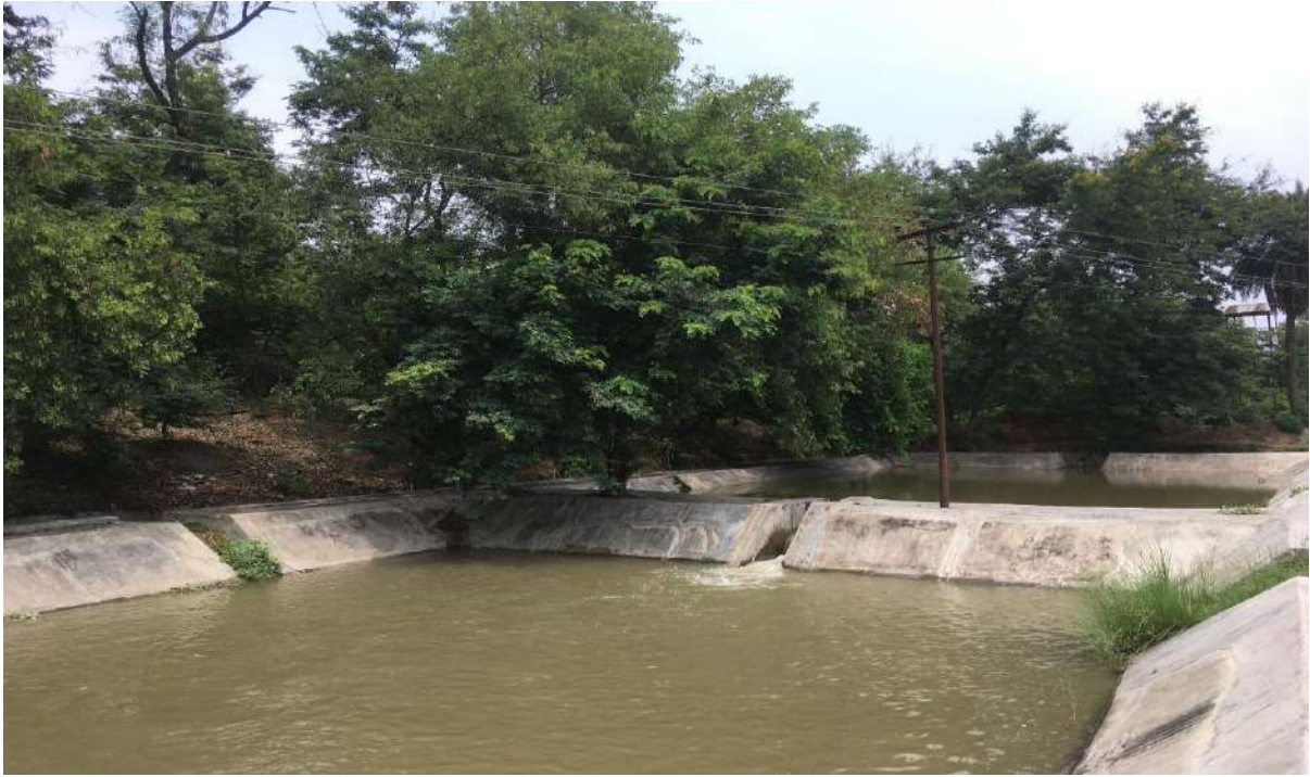
Photograph-6: Sedimentation tank
